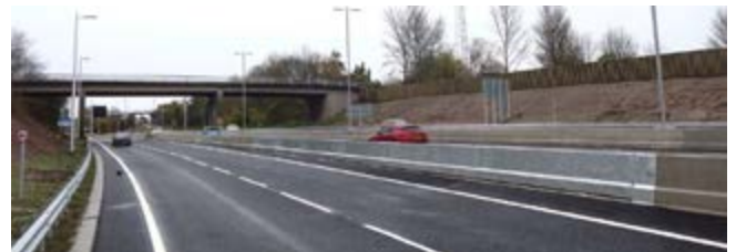
Steel Step Corridor
